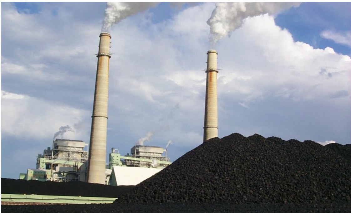
Smoke Stack from a Coal Fired Plant. Coal combustion produces 100 million tons of ash byproducts, such as bottom ash.
