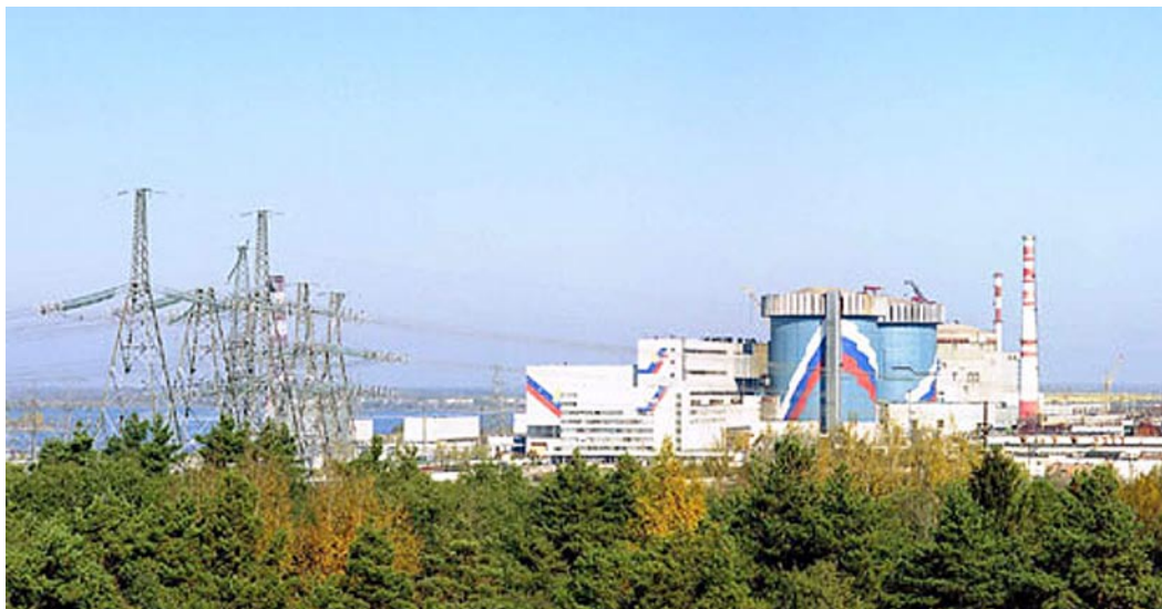
Kalinin Nuclear Power Plant, north of St. Petersburg (Russia).
